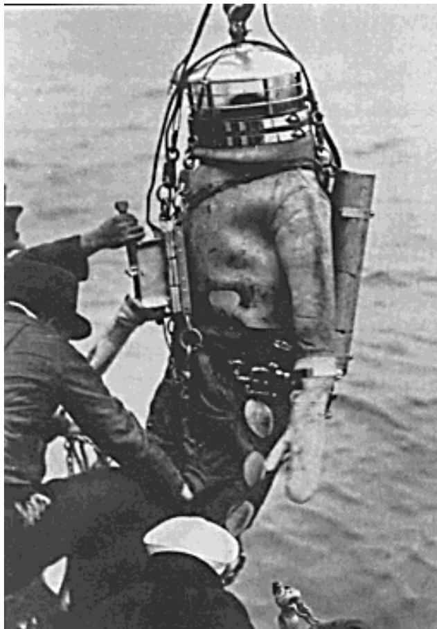
Max Nohl is lowered over the side of the *Antietam* to begin the dive. Note the braking device on the diver's chest to help retard his descent.
